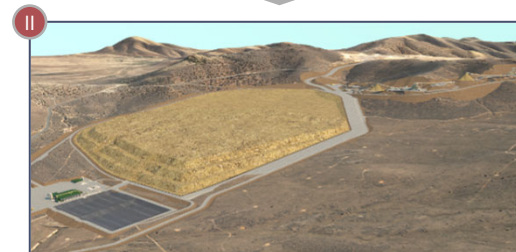
Stage VI leach pad (capacity of 300M tons)
